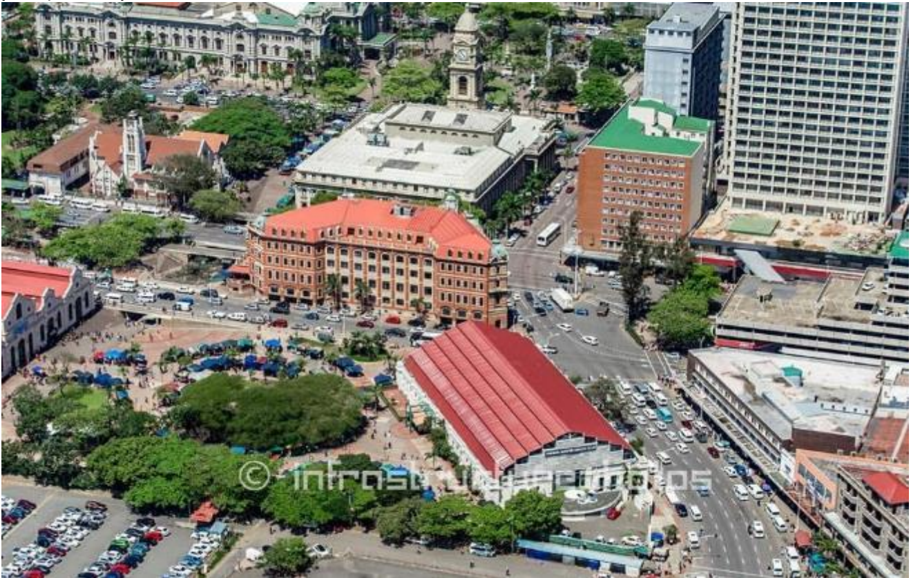
Figure 17: A bird's eye view of the south- western corner of the site with Workshop Retail Centre (to the far left of the photo) and the plaza with informal trader stalls.
